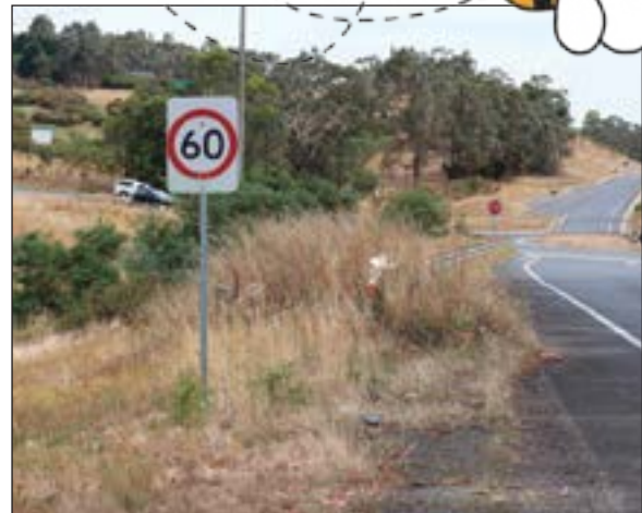
HIDDEN DANGERS: This grassy mound, located on the side of the northbound Hume Freeway Kilmore-Wandong off-ramp conceals hazardous items.
