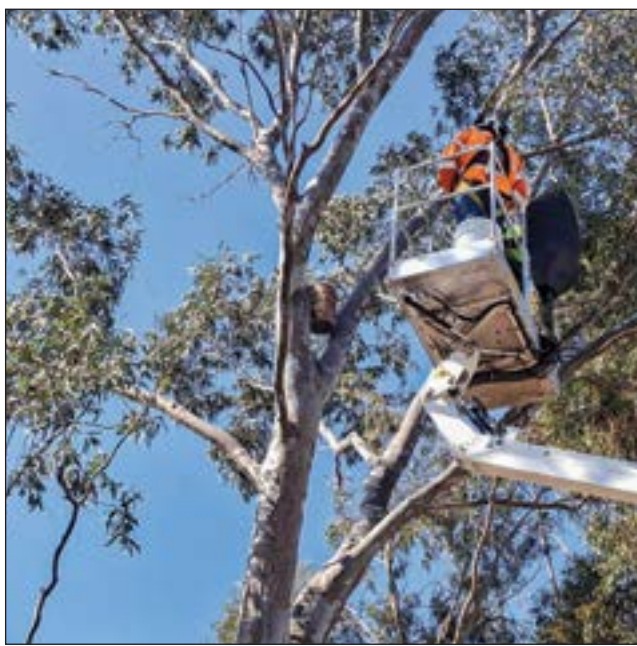
IN THE TREETOPS: A crane was used to install the hollows safely.
