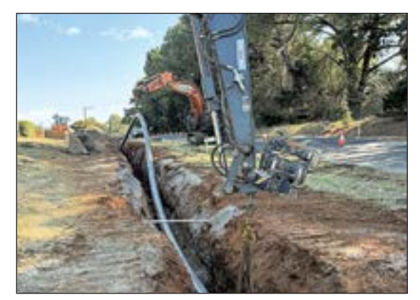
MIND THE GAP: Underground works in Lancefield have recently been completed.
